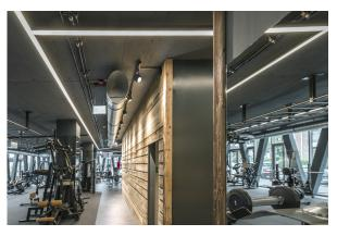
08 The PROLED L-Line Standard 24 aluminium profile is mounted directly on the reinforced concrete ceiling.
